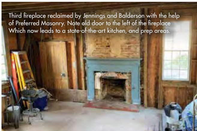
Tavern fireplace with rebuilt foundation in the Tavern room facing St. Margaret's School. Original brick was repointed in all the fireplaces, chimneys and hearths.
